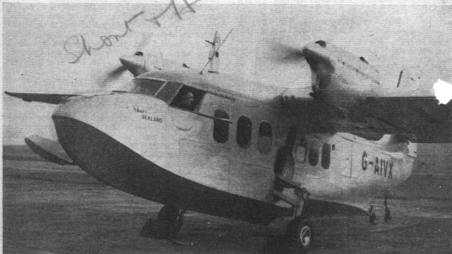
POWER CHECK : The two D.H. Gypsy Queen 70s, here seen running up, will soon lift this prototype Short Sealand amphibian on a first flight over the Belfast Lough. Reversible-pitch airscrews are fitted to these geared and supercharged "Queens" to aid in handling on the water.
