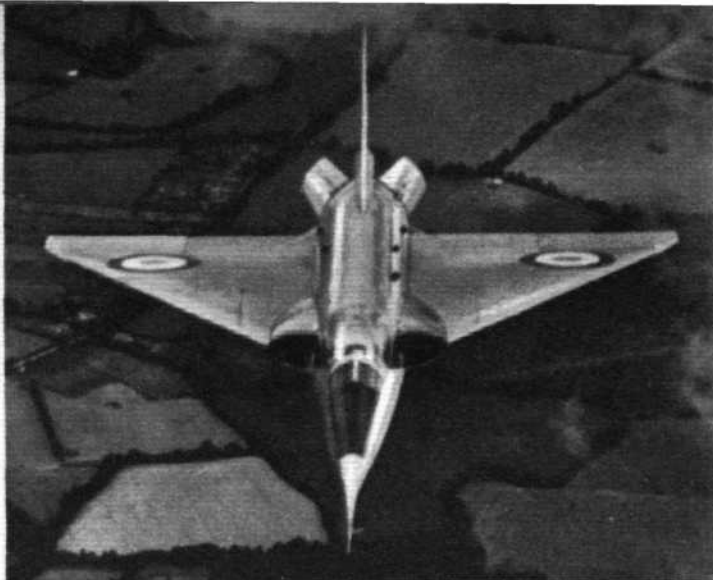
Points of interest in the "Flight" photograph of the Fairey F.D.2 (left) are the rear-fuselage air brakes and the small intakes atop the fuselage. The Sabre in the picture above is referred to in the paragraph headed "Canadair Sabre F.4."
