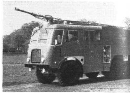
Sun fire/crash tender on Thornycroft chassis with Rolls-Royce engine
