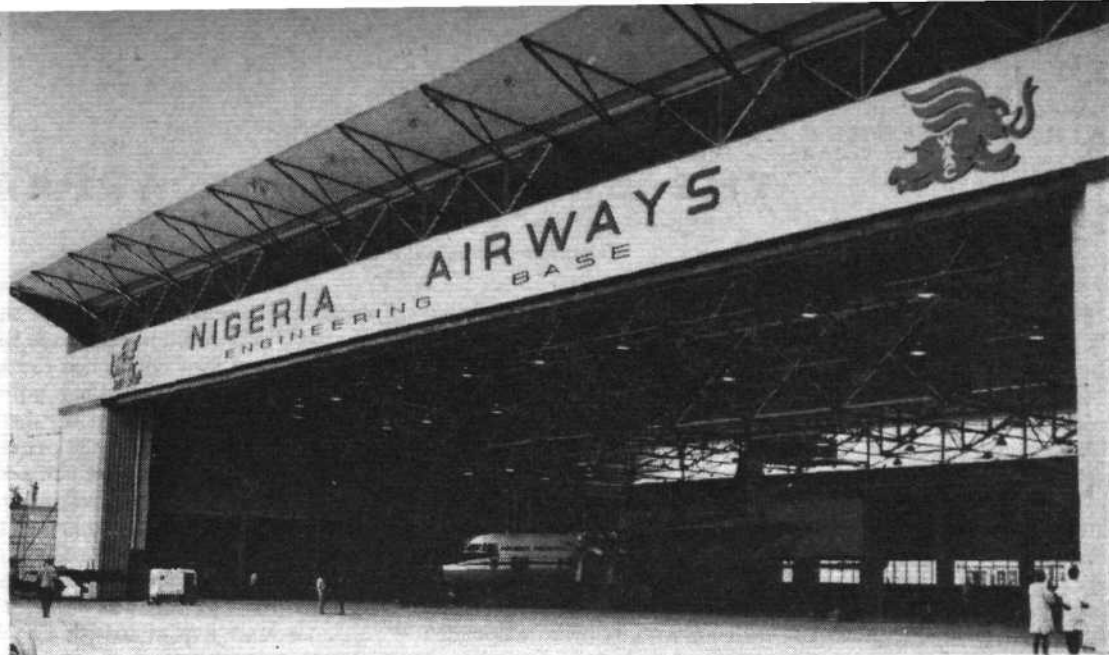
Nigeria Airways' fine new £900,000 engineering base at Lagos was opened by the President of Nigeria, Dr Nnamdi Azikiwe, on December 13. It incorporates an office block and a training school
