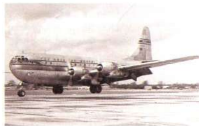
STRATOCRUISER: Boeing's 1947 Model 377 was the first widebody airliner
