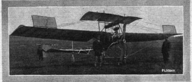
Front view of the aeroplane with which Mr. Eugene Gratz is experimenting at Canewdon, near Southend, to which reference has been made in these columns recently. This shows the general arrangement of the machine. The balancing flaps on the main planes are shown in their raised position.
