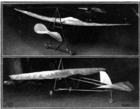
in position when gluing; tail plane is 12 ins., tapering to  $\frac{3}{4}$  ins. at rear. Total length, 33 ins. Motor power, 20 strands of  $\frac{1}{16}$  in. elastic, and Cochrane propeller (or tractor),  $8\frac{1}{2}$  ins.; the body of model is made of  $\frac{1}{4}$ -in. hardwood and aluminium rib wire.
