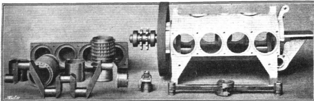
Fig. 3.—Some component parts of an 8-cyl. Ashmussen aero engine, as fitted to a Wright model B biplane.
