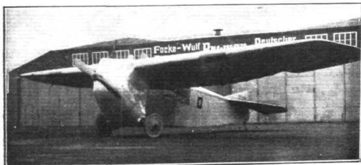
A development of the type A.16 is the Focke-Wulf A.16A, which has a 100 h.p. Mercédès engine. Yet another development is the A.16b, which is fitted with a Junkers L. 1a engine of 78 h.p.
