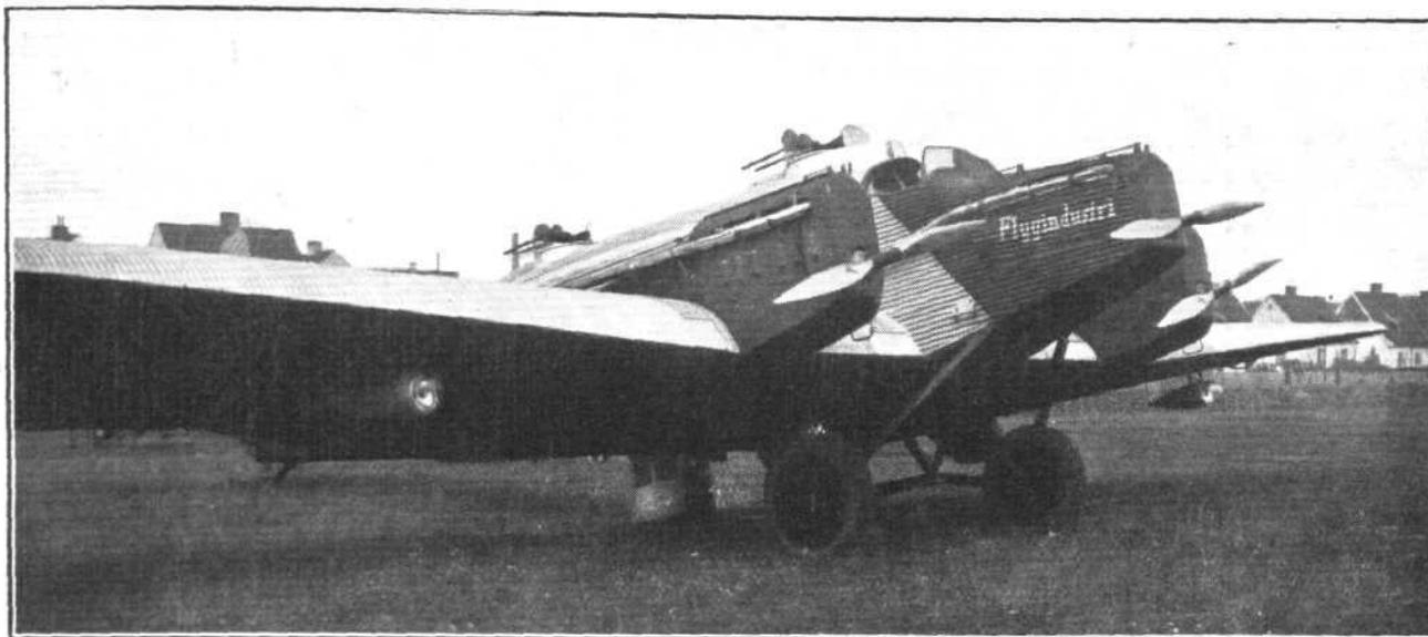
AT THE COPENHAGEN AERO SHOW: Three-quarter front view of the Junkers R.42 with three Junkers L.5 engines. This machine has been built by the Swedish Company A.B. Flygindustri, of Limhamn. Note the profusion of machine guns, and the gunners' turret under the machine.
