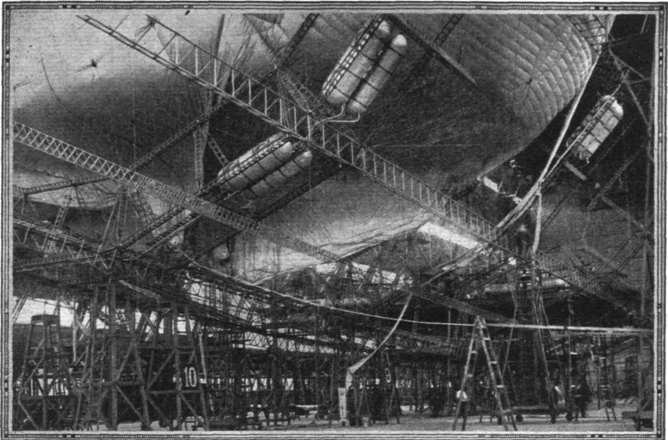
**R.101: Portion of the structure, before putting on the outer cover. Some of the gas bags may be seen in place. Note also the placing of the fuel tanks. ("FLIGHT" Photo.)**
