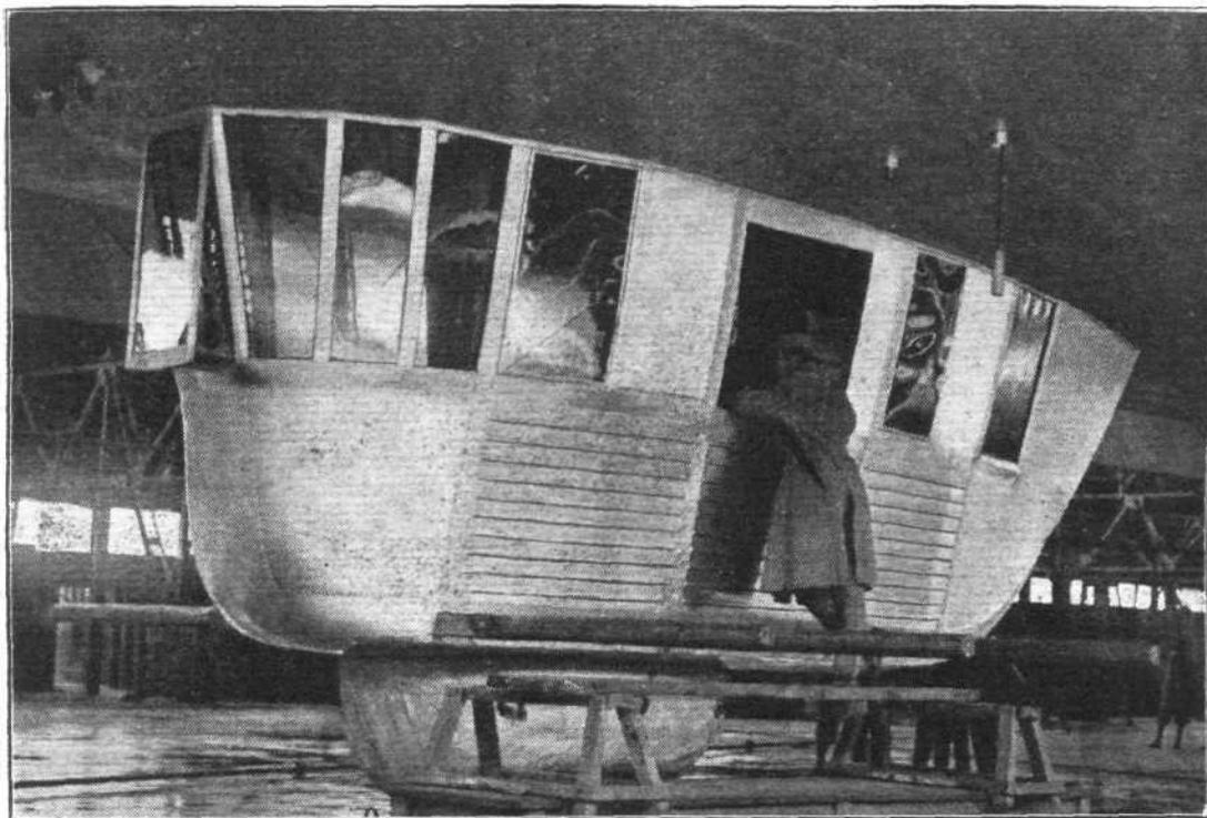
The Control Car of R.101 is quite a small affair, but the Captain's Control Room is immediately above it, inside the main hull.
