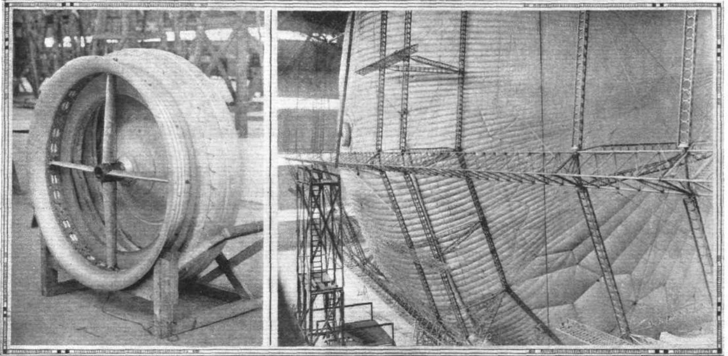
**SOME R.101 DETAILS :** On the left one of the gas valves, and on the right a portion of the structure. The main longitudinals are seen in place, but of the intermediate longitudinals short lengths only were attached when this photograph was taken last year.
