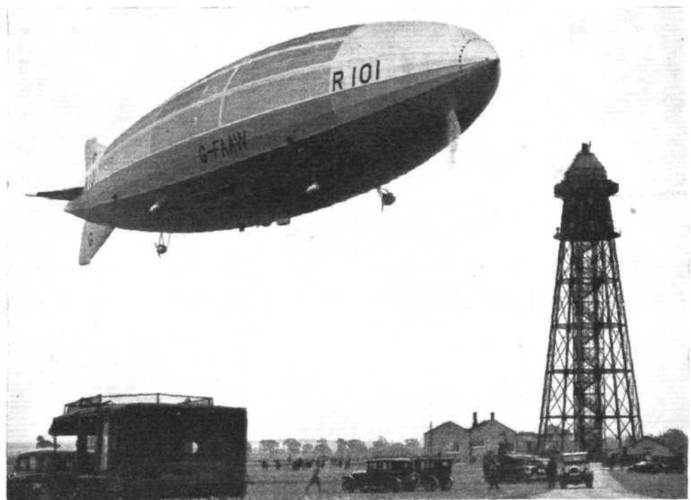
Three photographs which illustrate the beginning of the first flight of R.101 : The airship attached to the mast and, below, just cast off. Note the dropping of water ballast. (" FLIGHT Photos.")
