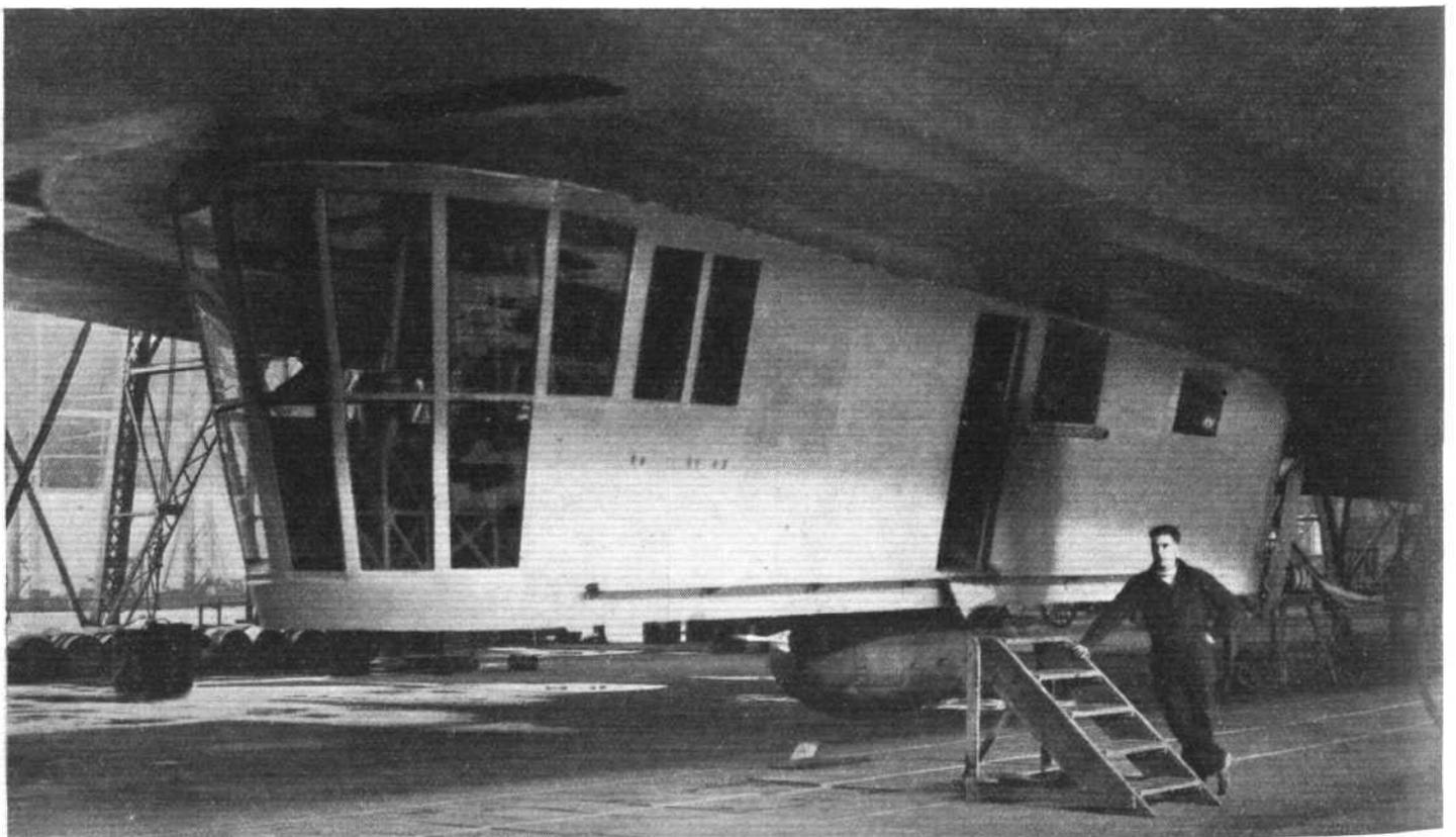
The control car of R 100. Note the bumper underneath. (FLIGHT Photo.)
