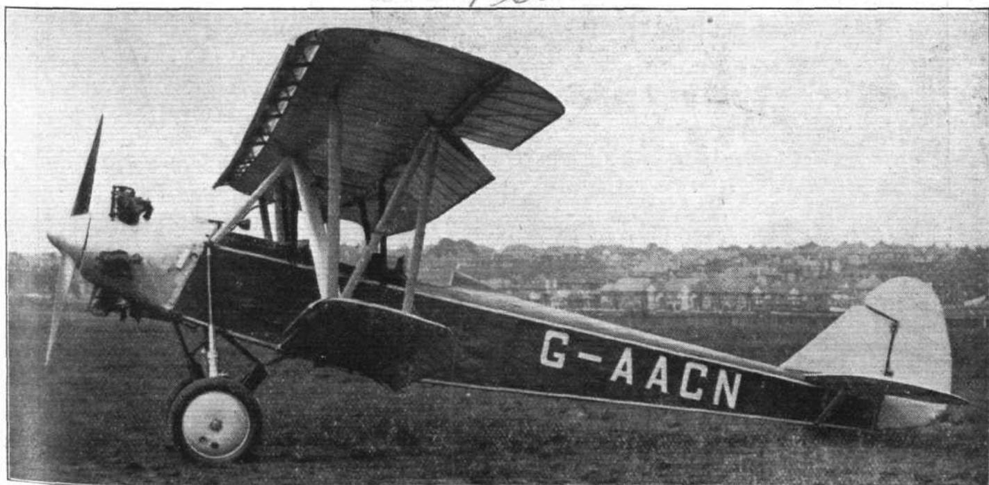
This side view of the Handley Page Guggenheim Competition machine shows very clearly the lift slots open and the trailing edge flaps down, in the position of maximum lift. (FLIGHT Photos.)
