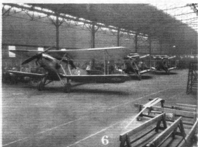
**TRACK ASSEMBLY OF AIRCRAFT AT BROUGH: (1) First stage, a "Ripon" fuselage on the track. (2) The next stage, the rear portion of the fuselage added. (3) Beginning of track, and "Ripons" in early stages of assembly. (4) "Ripons" nearing end of track; note overhead derrick. (5) "Ripons" nearing completion on the end of the track. (6) The final stages. In the foreground a "Ripon" ready for test flights.**
