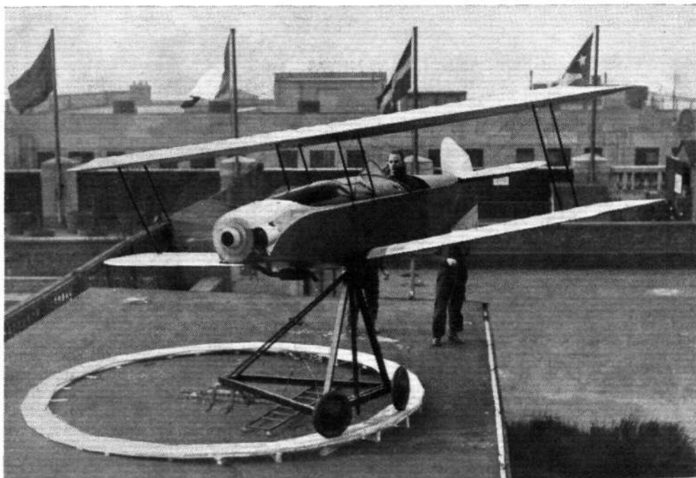
The Whitlet Hoverplane in its new guise as a biplane being flown on the roof of Selfridge's store in Oxford Street. This model answers to its controls much better than the original little monoplane and gives its users a truer idea of flying. (FLIGHT Photo.)
