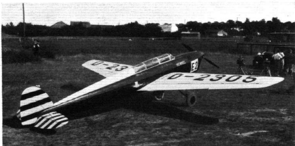
**GERMANY'S "WHITE HOPE":** The new Heinkel He. 64 ("Argus" engine) is characterised by a very slim fuselage and a longer lever arm for the tail than is usually found in German machines.
