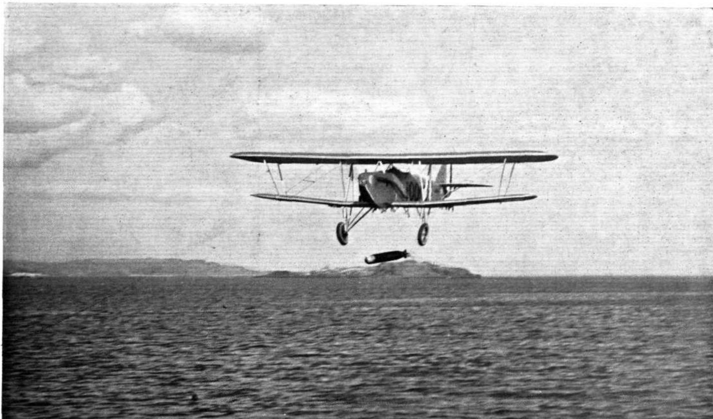
**DROPPING :** A "Horsley" after diving down to 15 feet from the surface discharges a dummy torpedo. The island of Inchkeith is in the background. (R.A.F. Official: Crown copyright reserved.)
