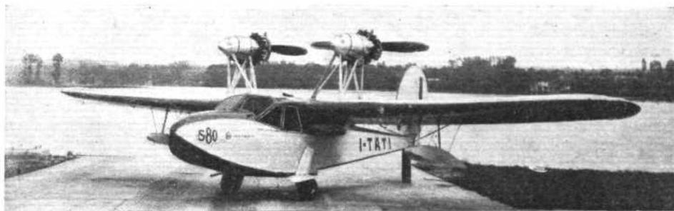
**BRITISH POWERED:** The latest Savoia-Marchetti S.80 four-seater amphibian, with two Pobjoy engines mounted as pushers. A maximum speed of about 122 m.p.h. is obtained.
