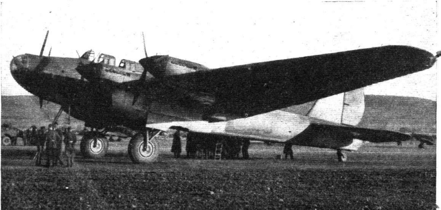
The Russian bomber in which Mr. Molotov flew to this country and to America. It appears to be roughly of the same dimensions as the Halifax and is powered by four liquid-cooled engines, which are probably of the 1,000 h.p. M-100 type. Another photograph of this machine appears on page 607.
