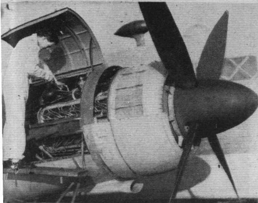
(Above) Warwick installation of the Napier Sabre VI with annular radiator. (Right) Graph showing performance at altitude of the Sabre VII on 100 octane fuel. \*Allows for drop in power due to weak mixture.
