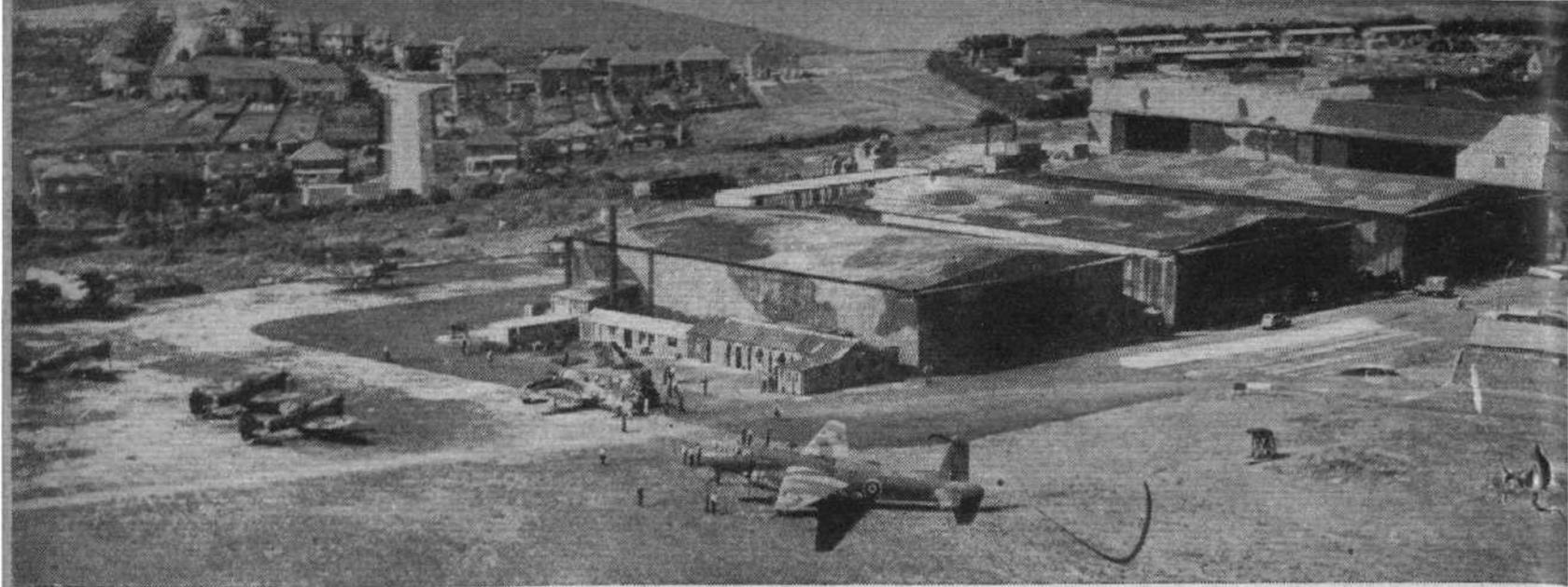
An aerial view of Napier's installation and flight-testing department at Luton airport. Engine-test aircraft can be seen on the tarmac. On the extreme left is a Manchester centre section used for engine testing.
