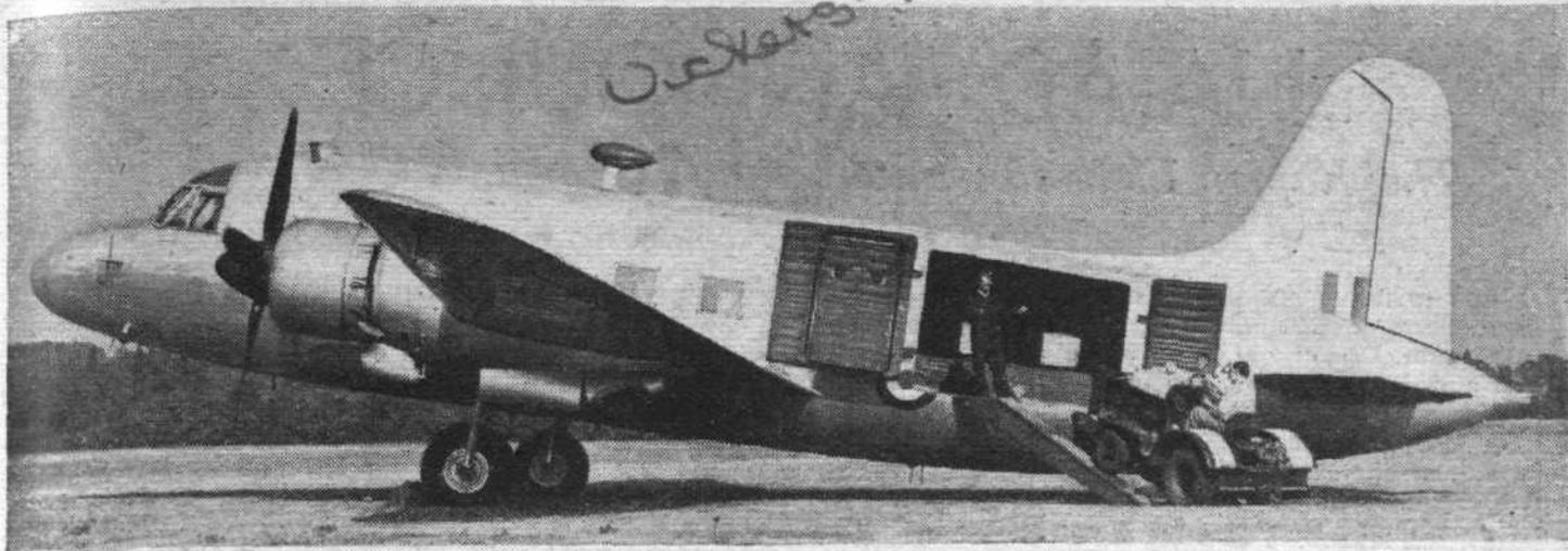
The Valetta C Mk I can be adapted for a number of transport duties. In freighter form, as above, the large double-entrance door makes possible the carriage of vehicles, guns, etc. An alternative load would be 36 troops.
