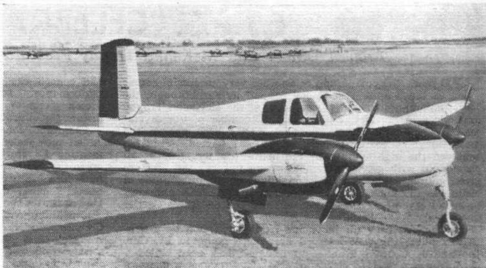
**BONANZA SENIOR**: The first photograph of the Beech Twin-Bonanza reveals a new design for an all-metal, 5-seat, light twin for the private or commercial owner. Powered by 260 h.p. Lycoming engines, the first Model 50, as it is designated, made its initial flights on November 15th. A cruising speed of over 180 m.p.h. and a range of 1,000 miles are among the estimated performance figures; six passengers can be carried with shorter-range fuel load. The price is estimated at 30,000 dollars.
