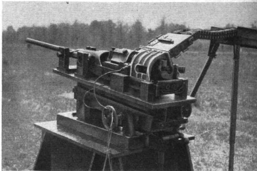
A development model M-39 on test, firing at long range in the open air. Points worth noting are the ammunition feed and electric ignition cable. The photograph was probably taken during 1952.
