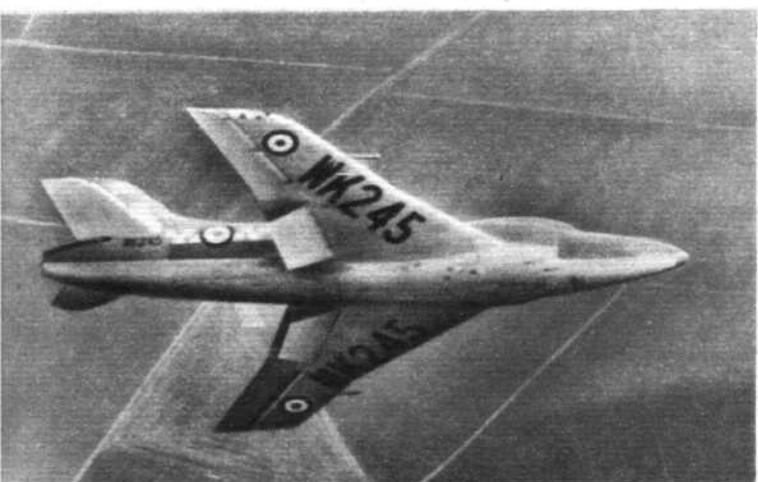
The second and last mark of Swift to reach No. 56 Sqn. was the Mk 2, here seen with four 30 mm cannon and kinked leading edge, but without saw-tooth wing, variable-incidence tail and afterburner as now standardized on the F.R.5.
