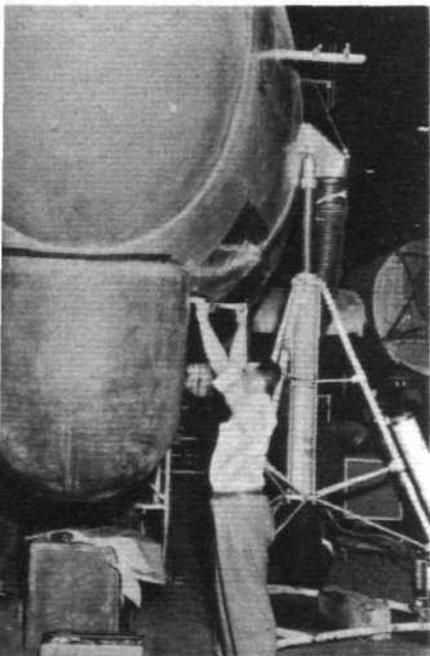
Above, new-type radome fitted to the 14th Argus; below, Sparrow 2 air-to-air missile, for which Canadair is co-ordinating contractor.
