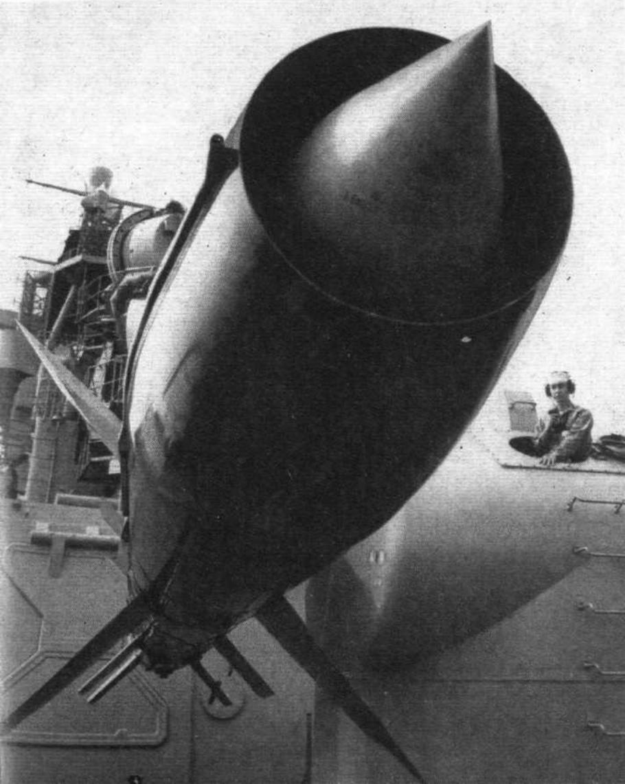
The nuclear Talos differs from h.e. rounds in having no semi-active homing system. It can be distinguished by the fact that no aeriels and sensing tubes mar the circumference of the intake
