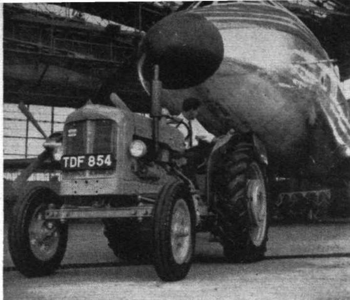
*Dowty have been developing hydraulic wheel drives for tractors for over two years. This Dowty Transmatic-equipped David Brown tractor was lent to the S.B.A.C. for the duration of the Show*
