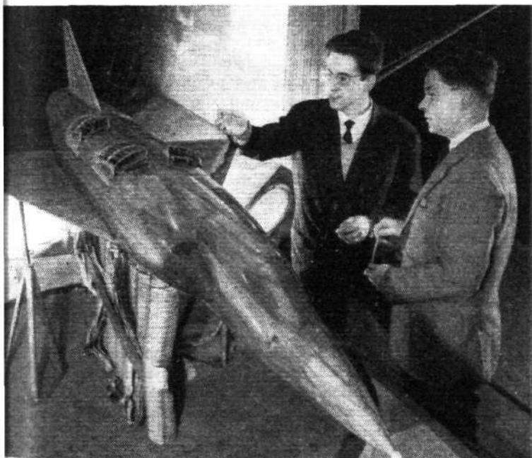
GAM Dassault have co-operated closely with Rolls-Royce in developing the Mirage IIIV, and in the picture above a lift-intake model of the big Mach 2 VISTOL strike fighter is seen in the 7ft by 5ft transonic tunnel at Hucknall. With it are M Fromantel (left), GAMD chief aerodynamicist, and Mr Conrad Bee of Hucknall's aerodynamics department. Both Dassault and Sud-Aviation have IIIV models on view (right)
