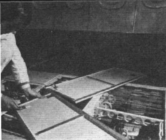
Integrally heated Thermolam flooring is fitted to the Hawker Siddeley Trident 2Es being delivered to BEA. Manufactured by Palmer Aero Products Ltd, the flooring provides positive insulation between the passenger cabin and the unheated freight compartment. A heating element is incorporated under the upper skin of standard Aerolam.
